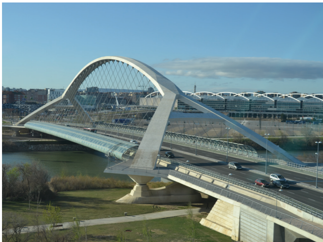
Third Millenium Bridge, Zaragoza, Spain, 2008 design: Arenas & Asociados structural design: Arenas & Asociados
